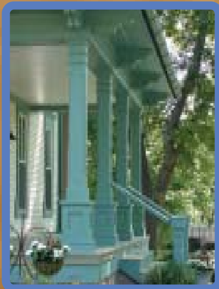
Custom square columns with raised panel pedestal base Photo courtesy of Brian Pennings
