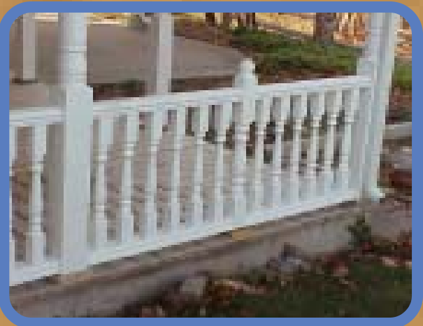
Shown are B4 baluster, TR2 Top rail, BR2 Bottom rail and NP4 3-1/2" colonial newel post
