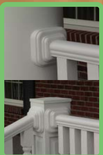
Custom mounting blocks for railing installation. Upper photo is a custom mount on a round column
